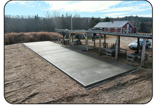
The new Pavillion foundation
